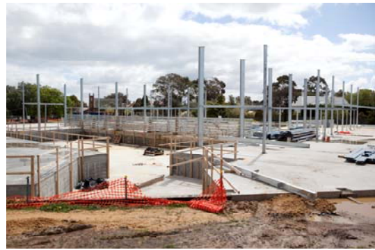
The multi-purpose hall at Bellarine Campus takes shape.
